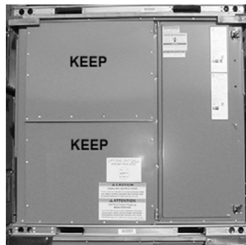
Figure 18: Save Side Panels For Economizer Hood Tops
