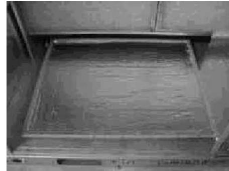
Figure 16: Return Downflow Plenum With Panel
